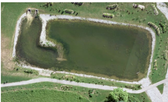
Stormwater Management Facility
