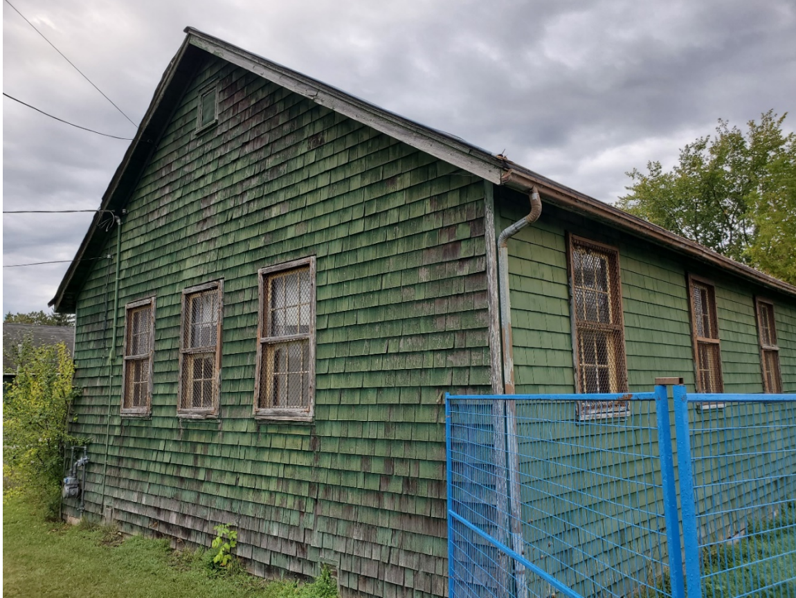
Figure 3: South and east façades of the former Canteen Building (looking northwest)
