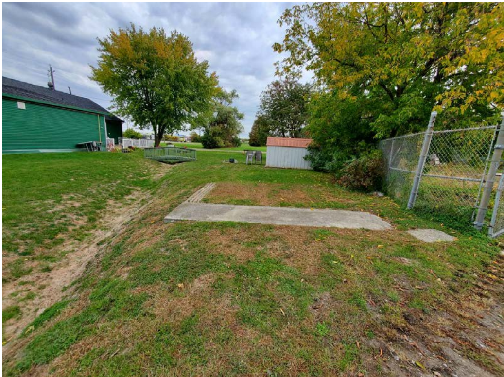
Figure 13: No. 10 Building, southeast façade and rear yard area (looking northeast)
