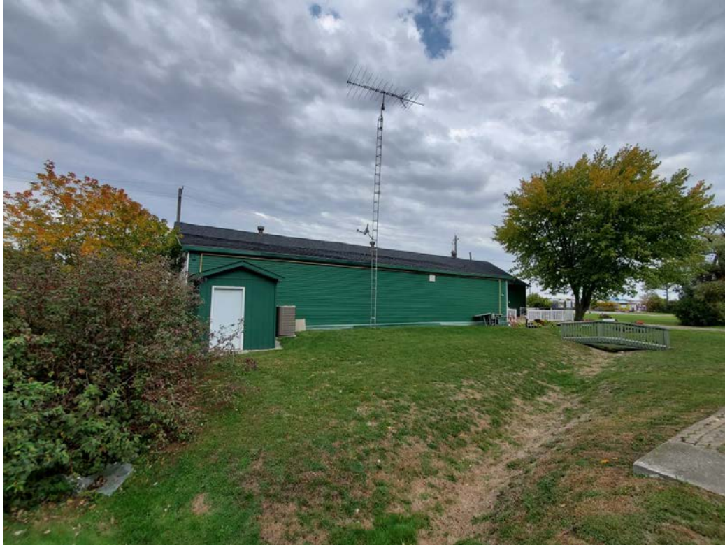
Figure 12: No. 10 Building, southeast façade (looking north)
