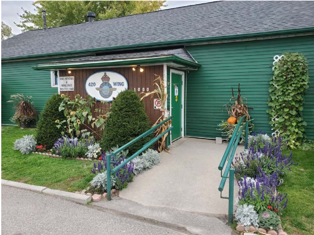
Figure 8: No. 10 Building, northwest façade (looking east), front entry
