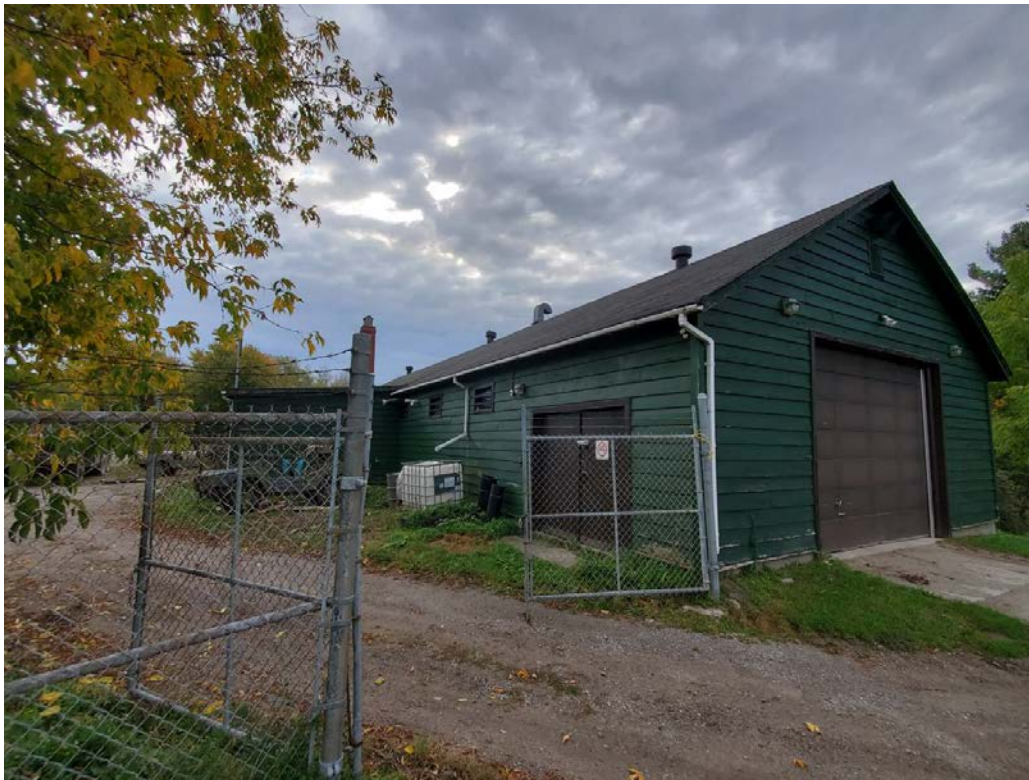
Figure 33: Former Stores Building, northwest façade, northeast facade and tank storage entry (looking southeast)
