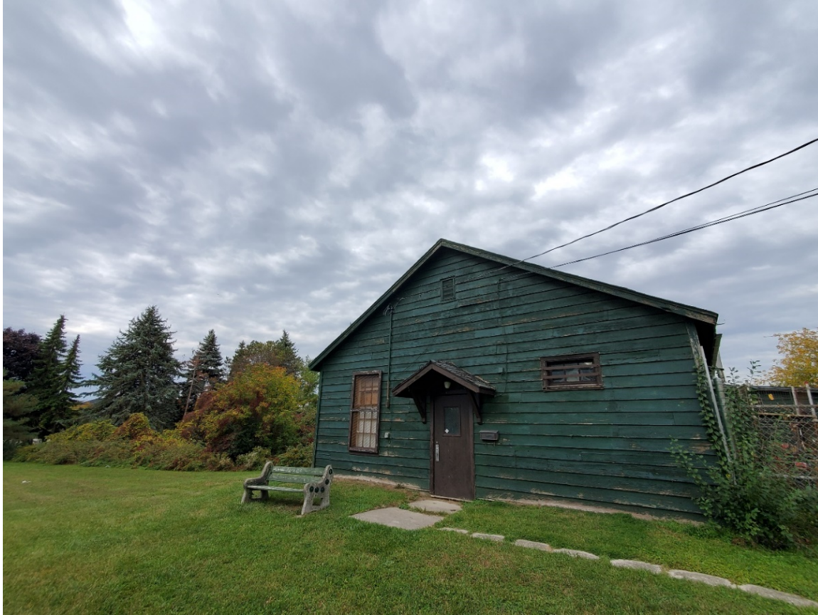
Figure 2: Front (south) facade of the former Stores Building (looking north)
