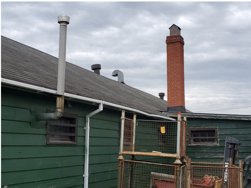
Figure 23: Former Stores Building, northeast façade (looking southwest), window detail
