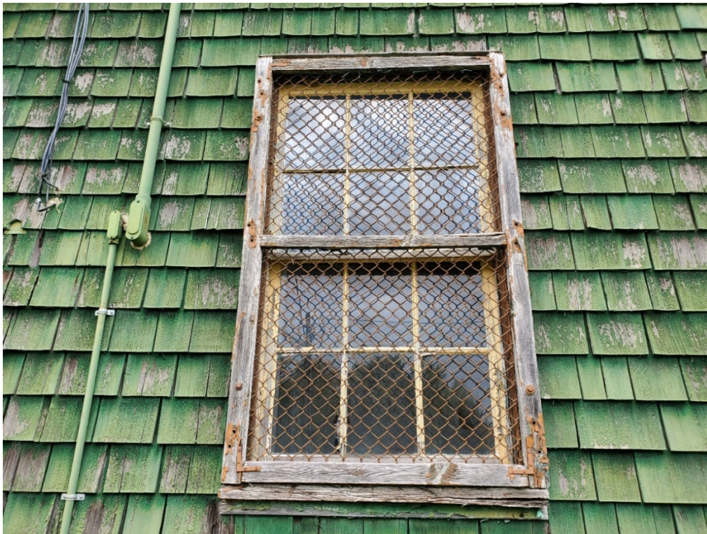
Figure 19: Former Canteen Building, southeast façade (looking northwest), window detail
