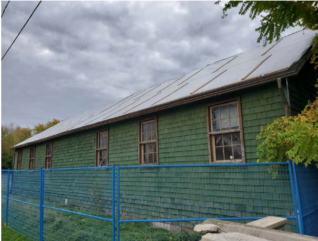
Figure 14: Former Canteen Building, northeast façade (looking south)
