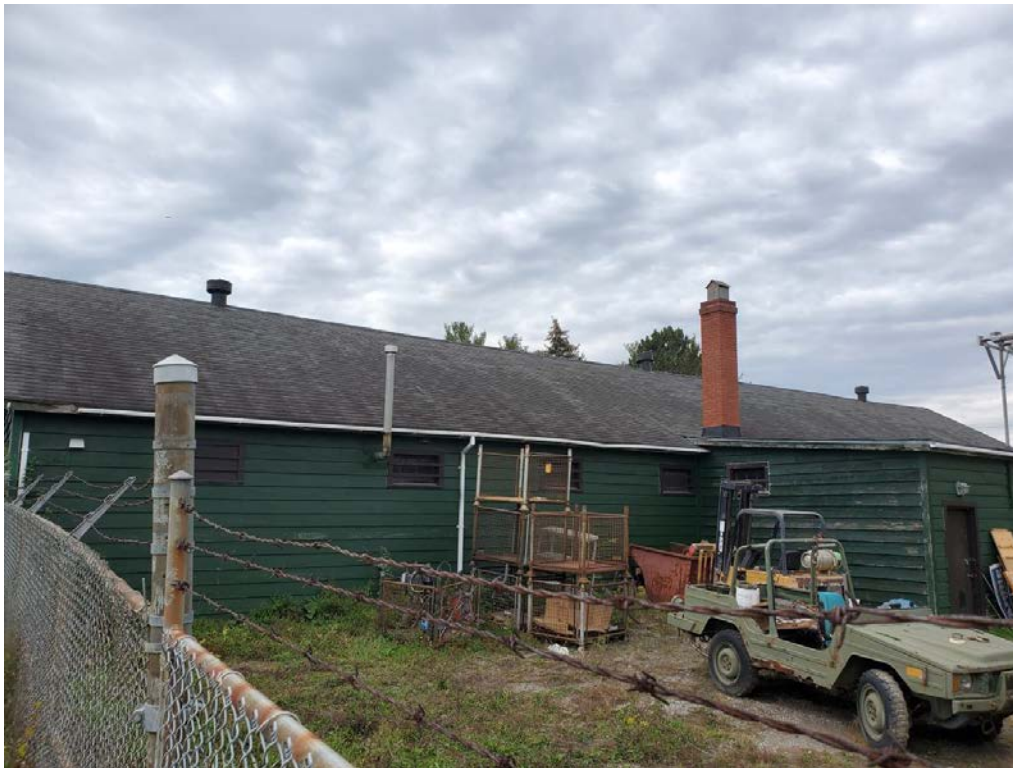
Figure 21: Former Stores Building, northeast façade and tank storage area (looking southwest)
