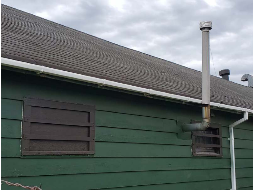
Figure 22: Former Stores Building, northeast façade (looking southwest), window detail
