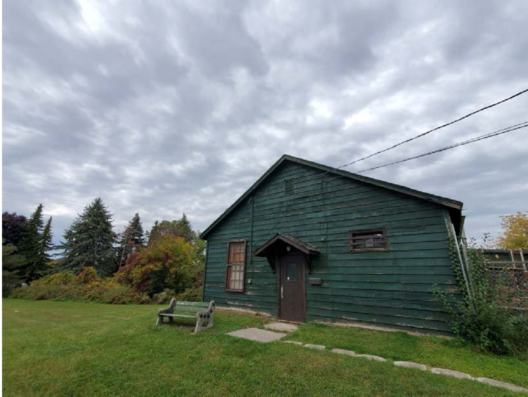
Figure 24: Former Stores Building, southeast façade (looking west), Airmen's Park to left
