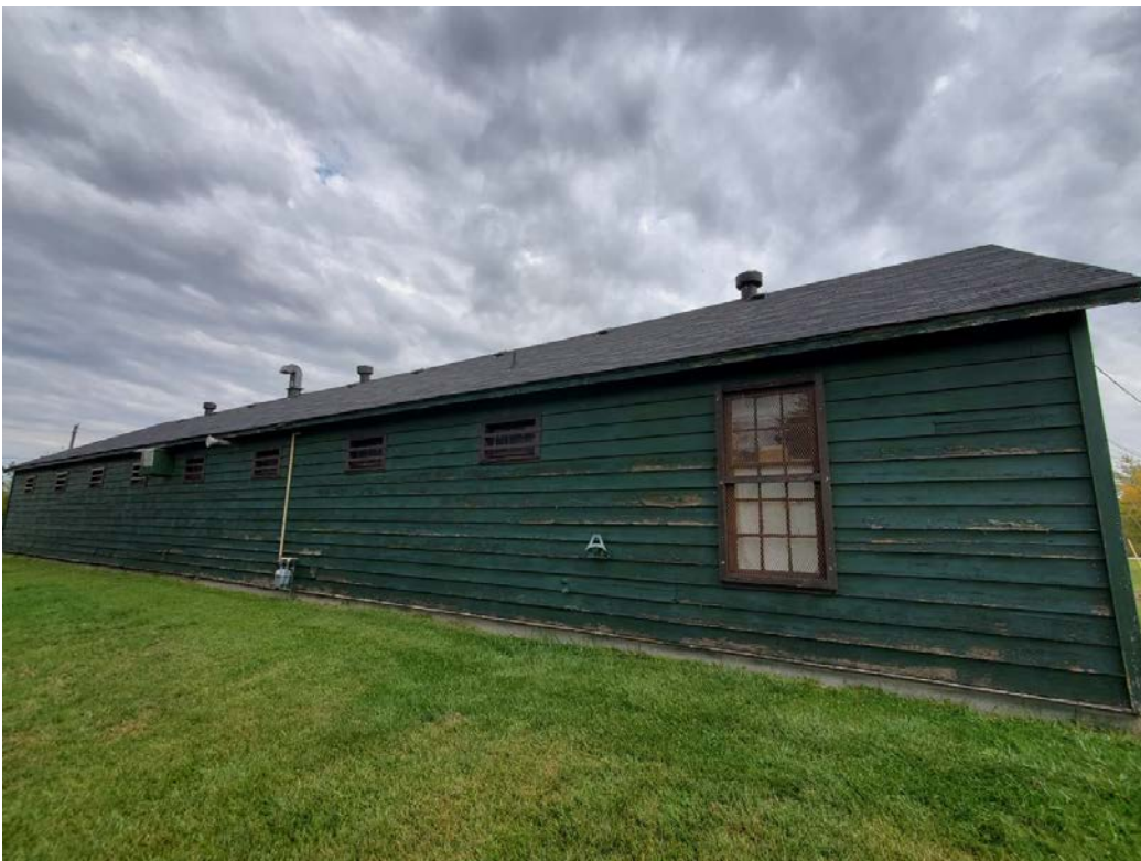
Figure 29: Former Stores Building, southwest façade (looking northeast)
