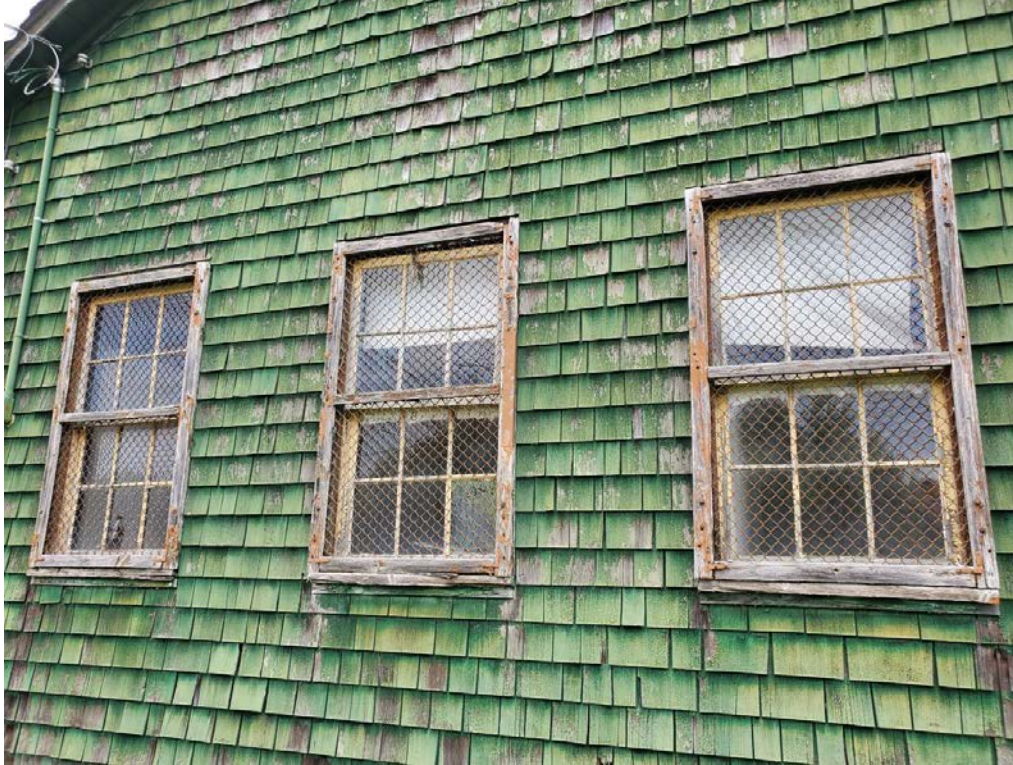
Figure 18: Former Canteen Building, southeast façade (looking northwest), window detail
