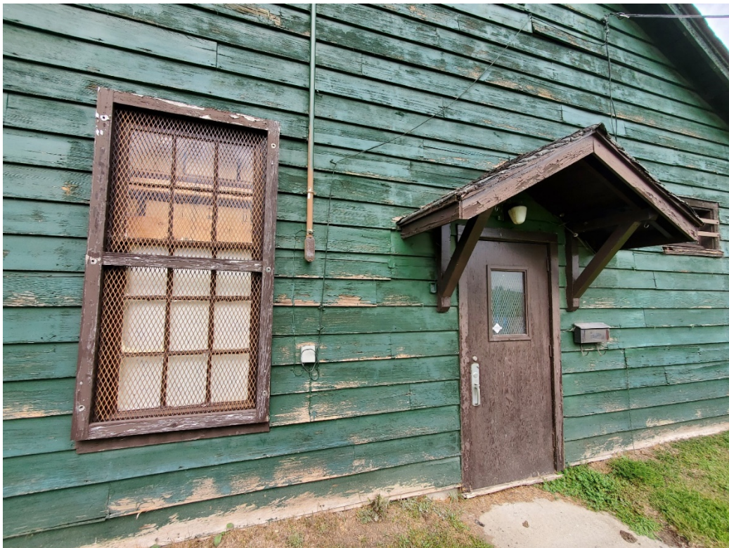
Figure 25: Former Stores Building, southeast façade (looking northwest), front entry
