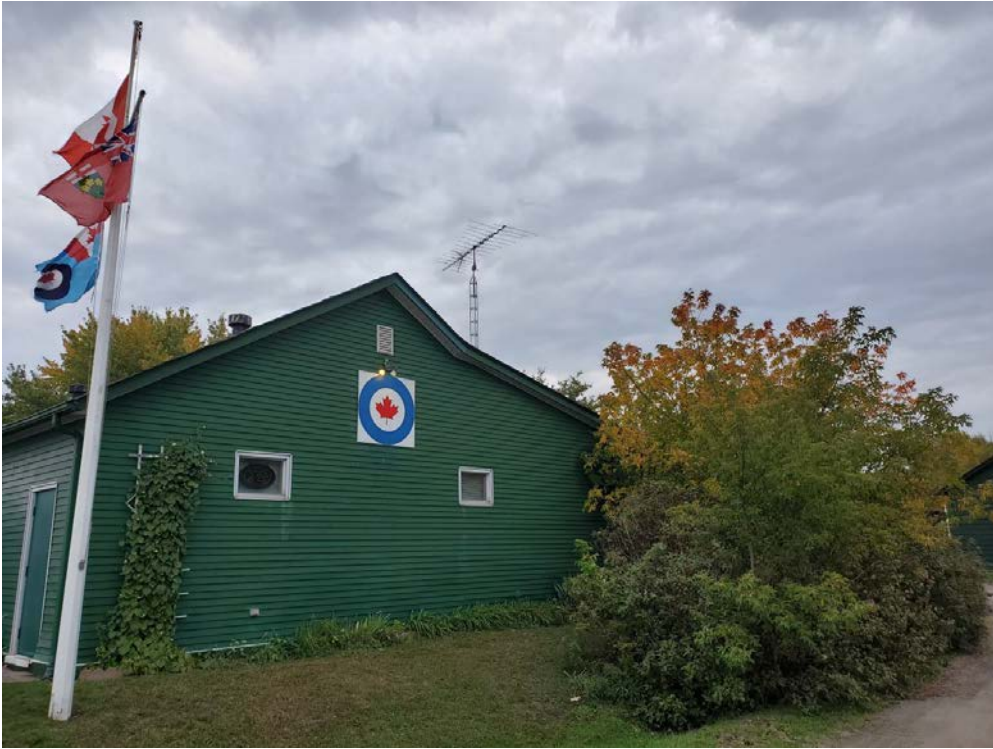
Figure 6: No. 10 Building, southwest façade (looking northeast)
