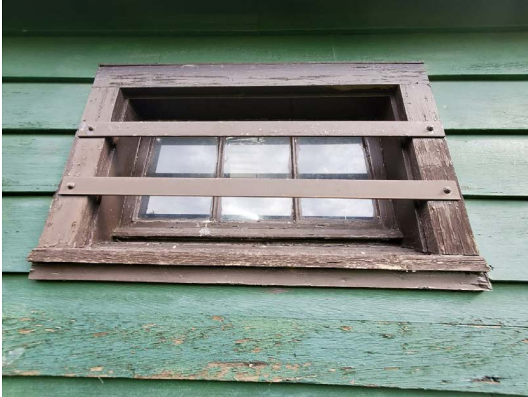
Figure 30: Former Stores Building, southwest façade (looking northeast), window detail
