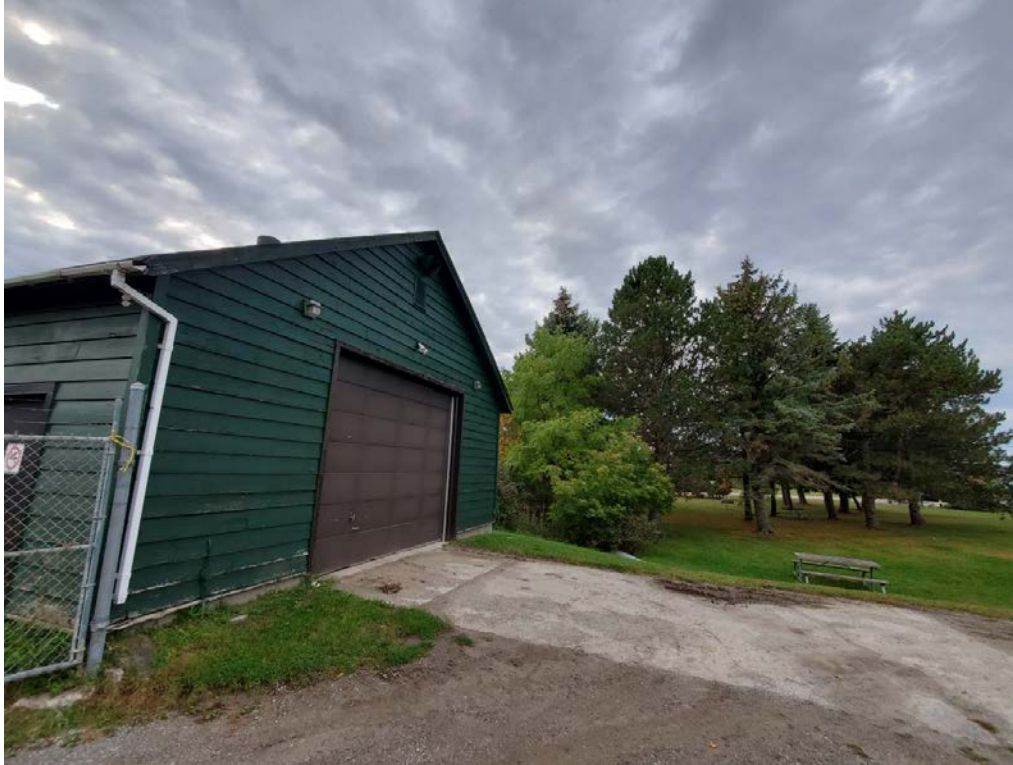
Figure 32: Former Stores Building, northwest façade (looking south), Airmen's Park to right
