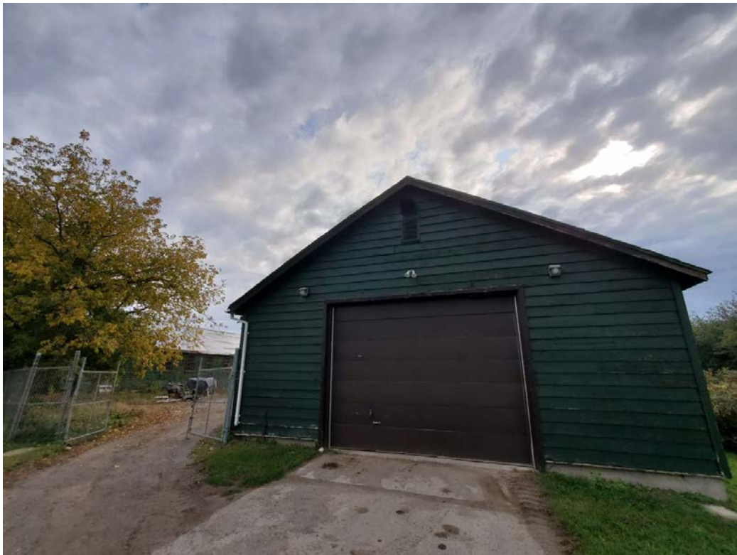
Figure 31: Former Stores Building, northwest façade and tank storage entry (looking east)
