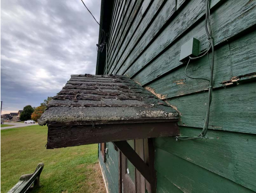
Figure 26: Former Stores Building, southeast façade (looking southwest), front entry canopy detail
