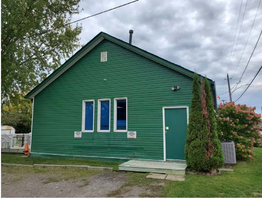
Figure 10: No. 10 Building, northeast façade (looking southwest)
