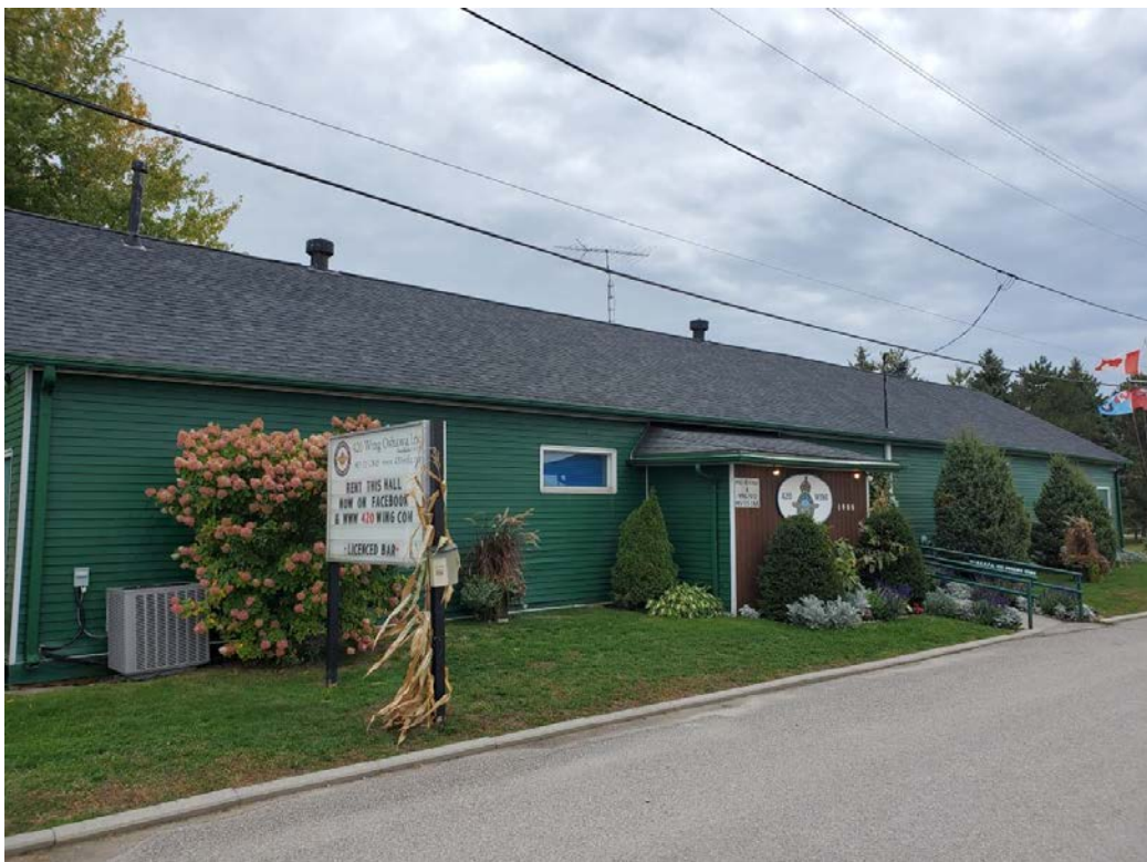
Figure 9: No. 10 Building, northwest façade (looking southeast)
