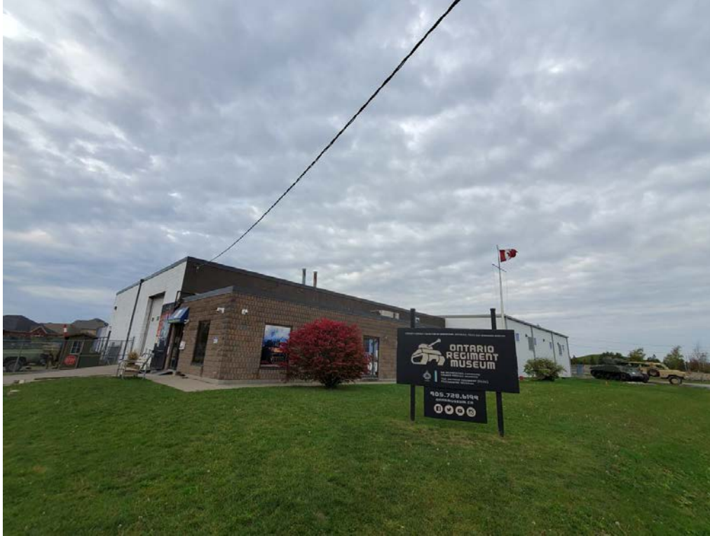
Figure 54: Ontario Regiment Museum (looking southwest) viewed from Stevenson Road North
