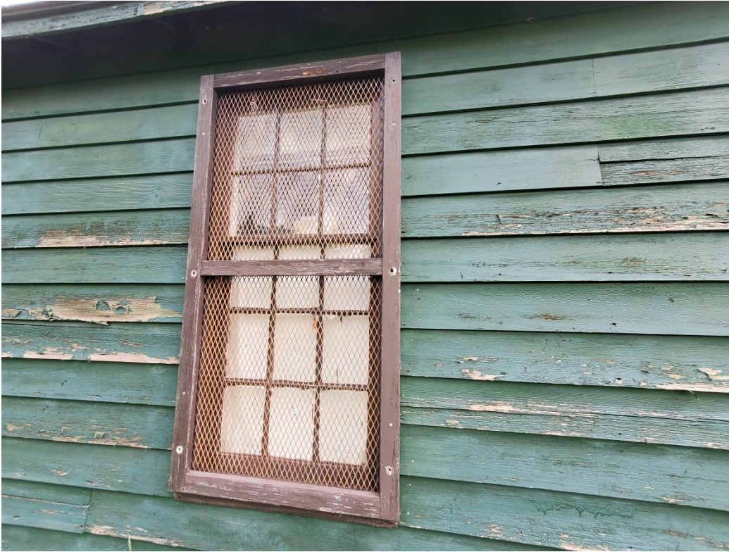
Figure 28: Former Stores Building, southwest façade (looking north), window detail
