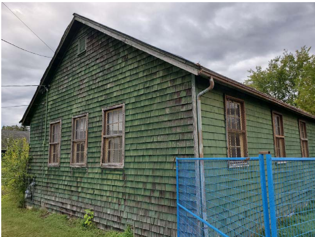
Figure 17: Former Canteen Building, northeast and southeast façade (looking west)
