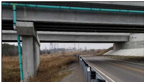
Figure 22: View of the Highway 407 East overpass
