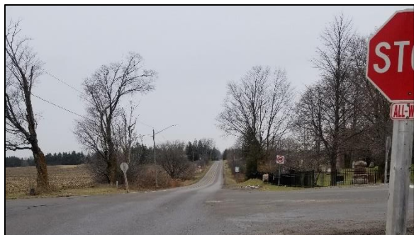
Figure 18: View of the intersection at Columbus Road West and Thornton Road North, facing east.
