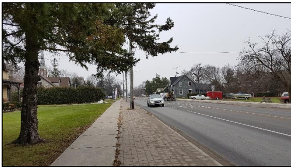
Figure 17: View to the south of Columbus Road on Simcoe Street North
