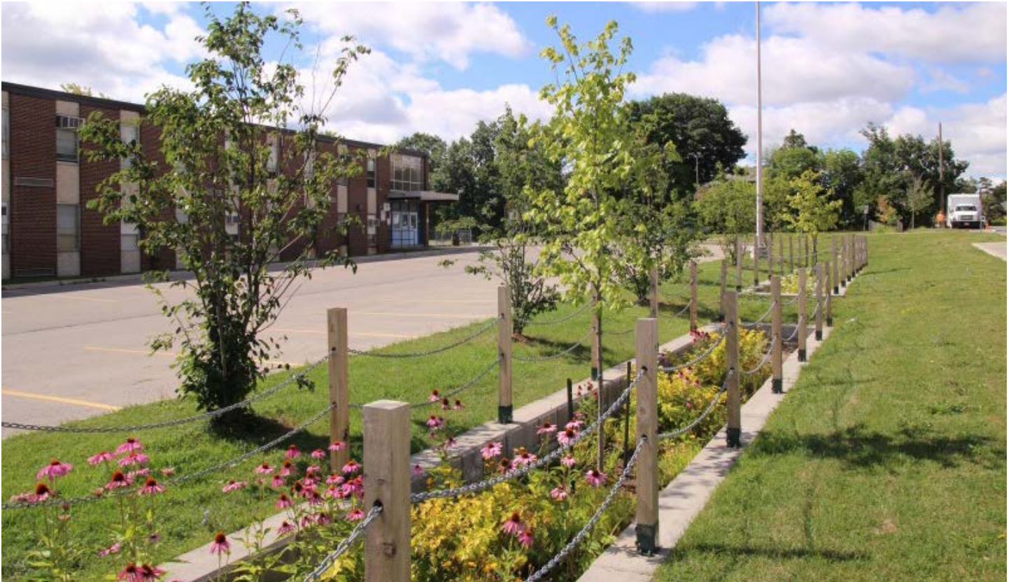
Rain gardens are bioretention areas that help manage stormwater (Water Canada).
