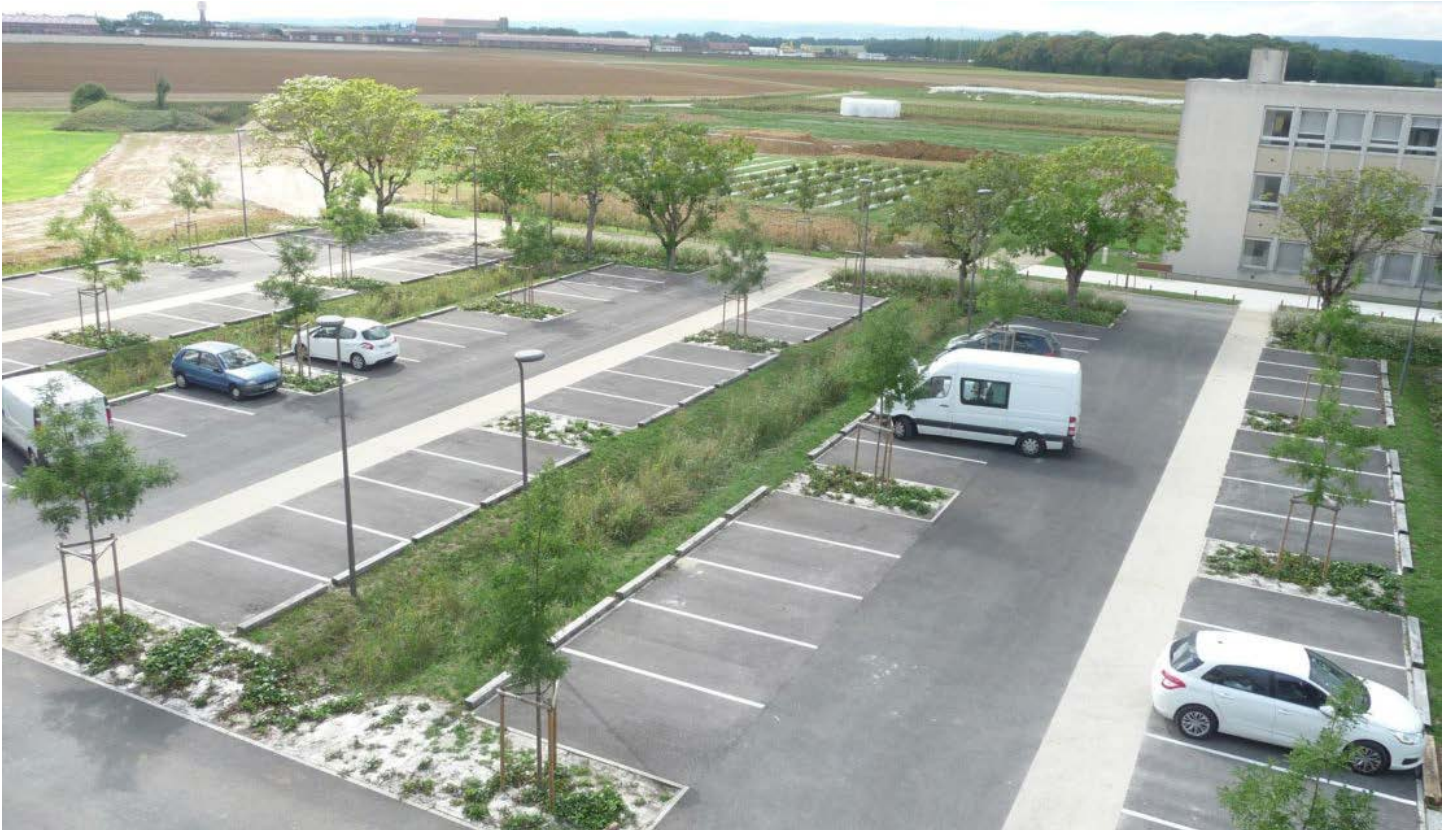
The surface parking lot above includes bioswales and tree plantings to improve stormwater management (Mayot & Toussaint Paysagistes).
