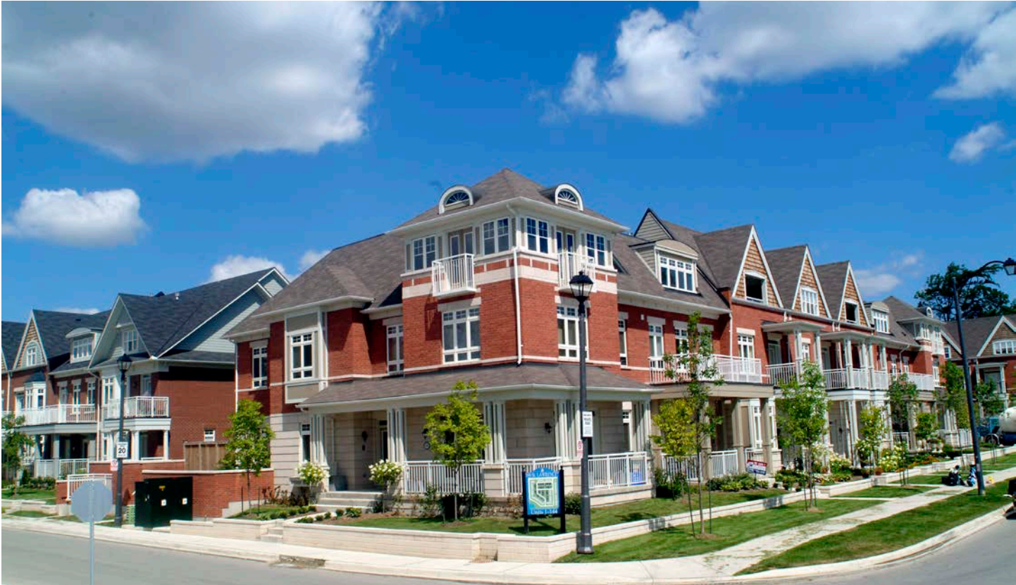
Buildings on corner sites should address each street edge with a design that addresses the existing street character and patterns (Brook McIlroy).
