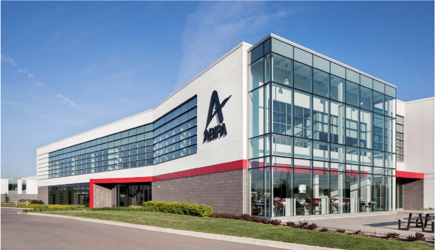
An employment building with signage integrated into the building design (GKC Architects).
