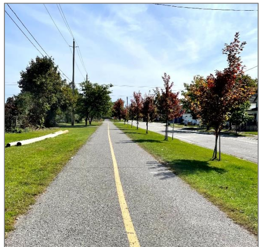
FIGURE 2-2: MICHAEL STARR TRAIL ADJACENT TO FRONT STREET
