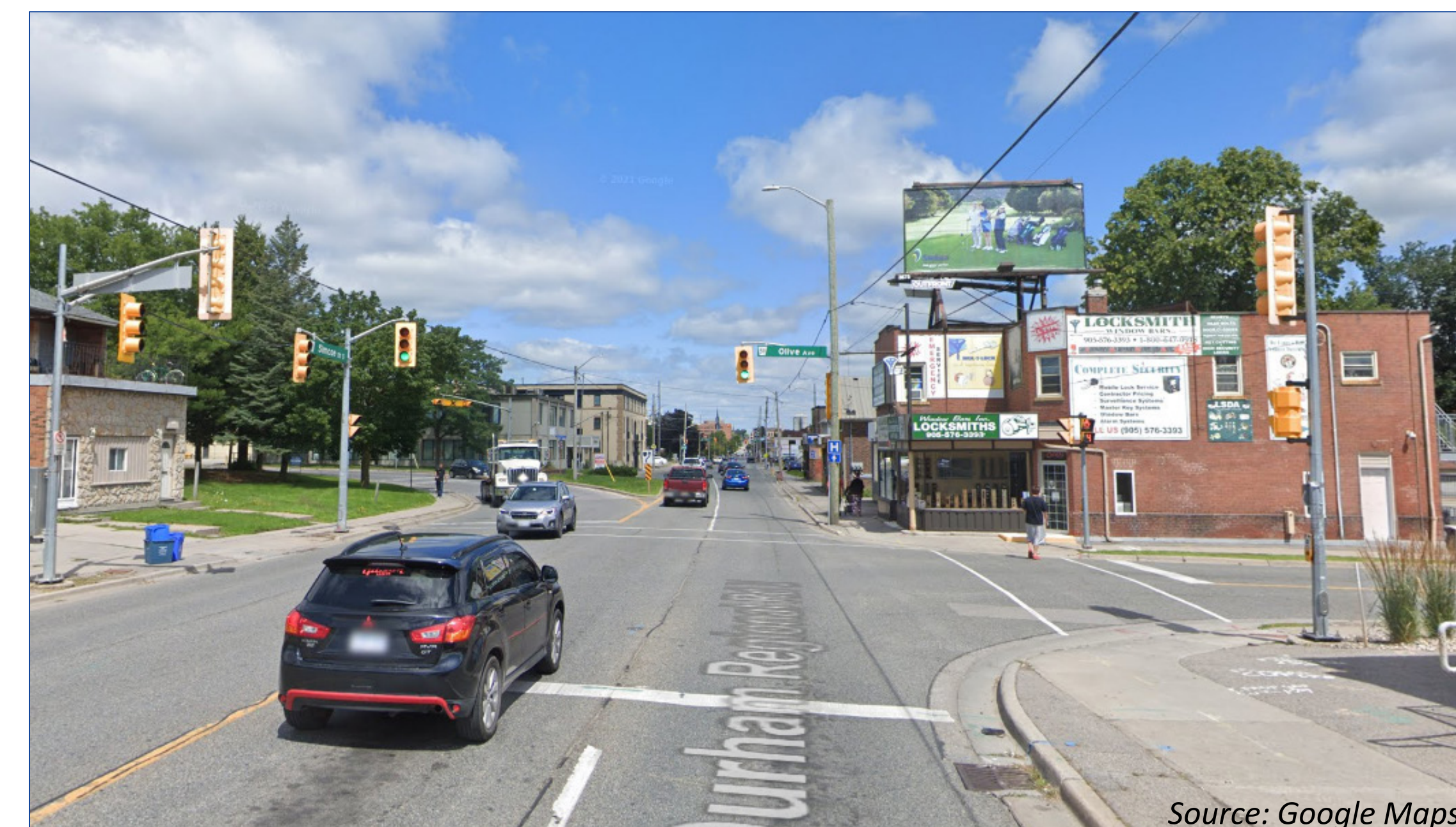
Intersection at Olive Avenue and Simcoe Street South, Oshawa
