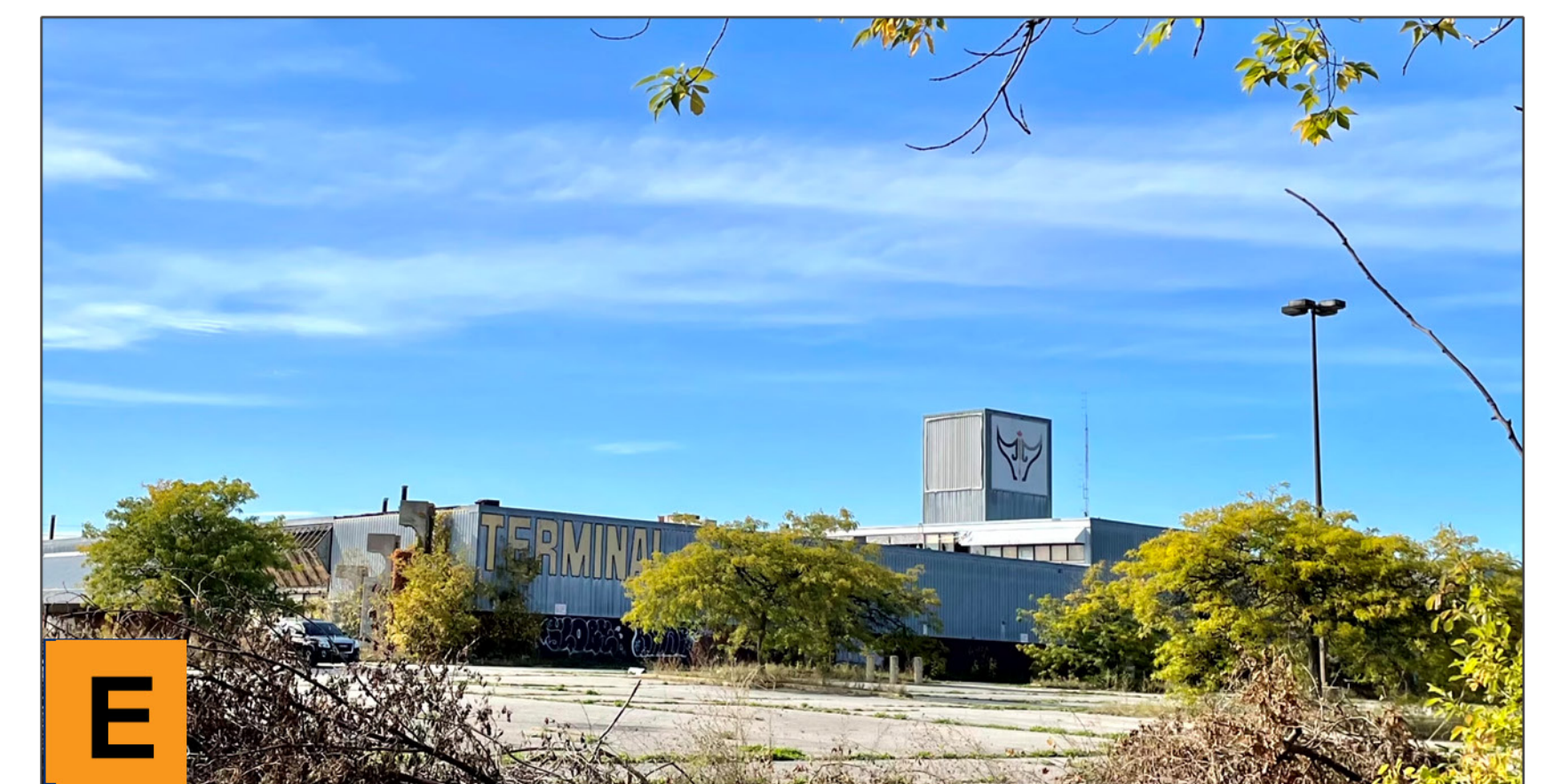
E Former Knob Hill Terminal, Oshawa
