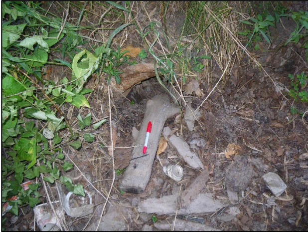
Upstream end of culvert facing downstream (west). Note small size and very dry characteristics.
