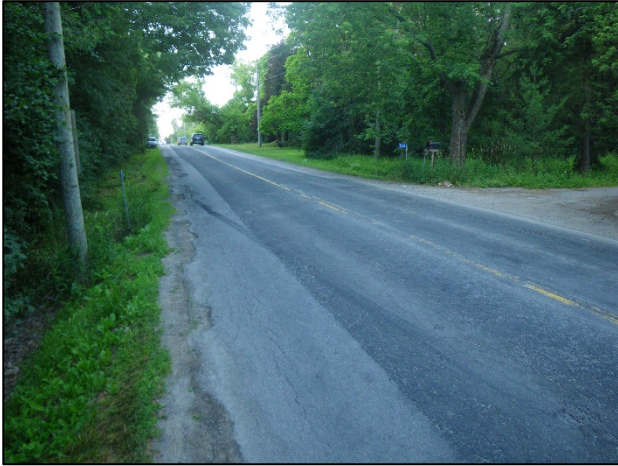
Facing south at Crossing 1. Note there is no "dip" in the road indicating a lack of a valley or floodplain.
