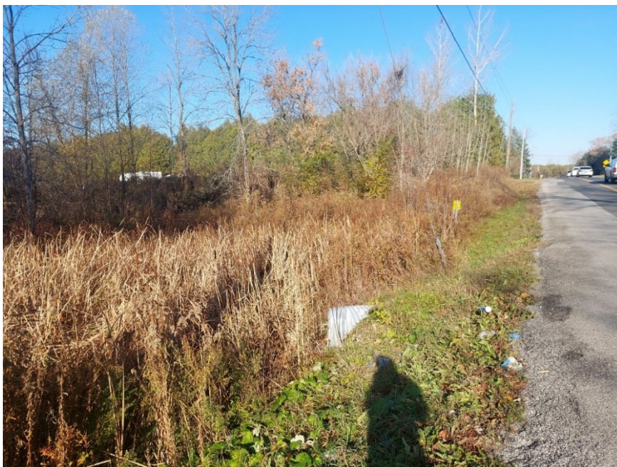
Plate 8: View of the culvert and floodplain of the stream, looking north (A.S.I., 2022).
