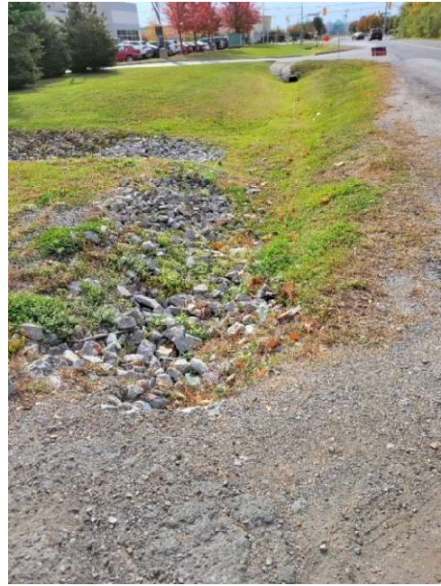
#8-C3 looking south
