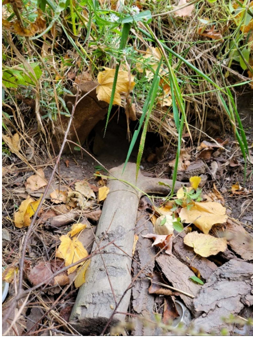
#1- Centerline Culvert 1, outlet
