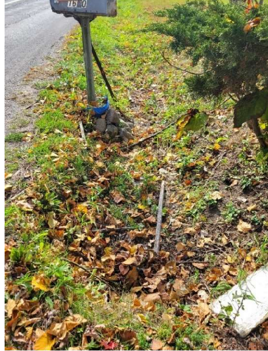
#58-C16 Looking south
