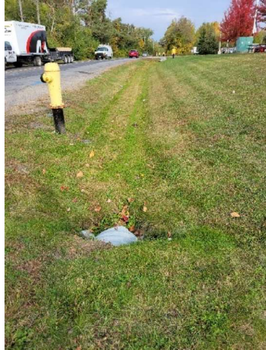
#2-C1 looking south
