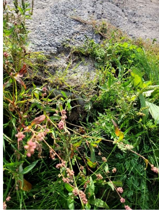
#81-C22 Looking south
