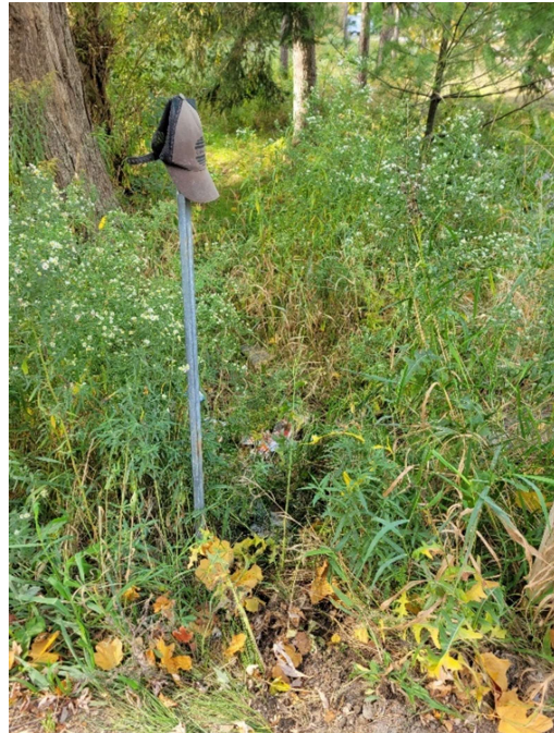
#4- Centerline Culvert 1, looking west
