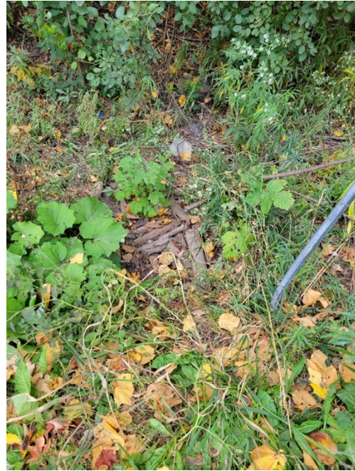
#2- Centerline Culvert 1, looking east
