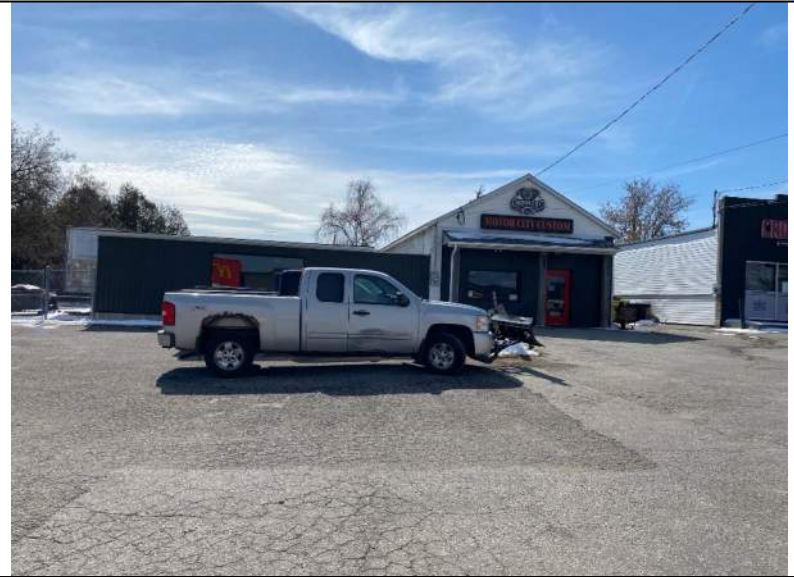
Photograph 10: View looking south at vehicle repair garage at 287 Dean Ave.
