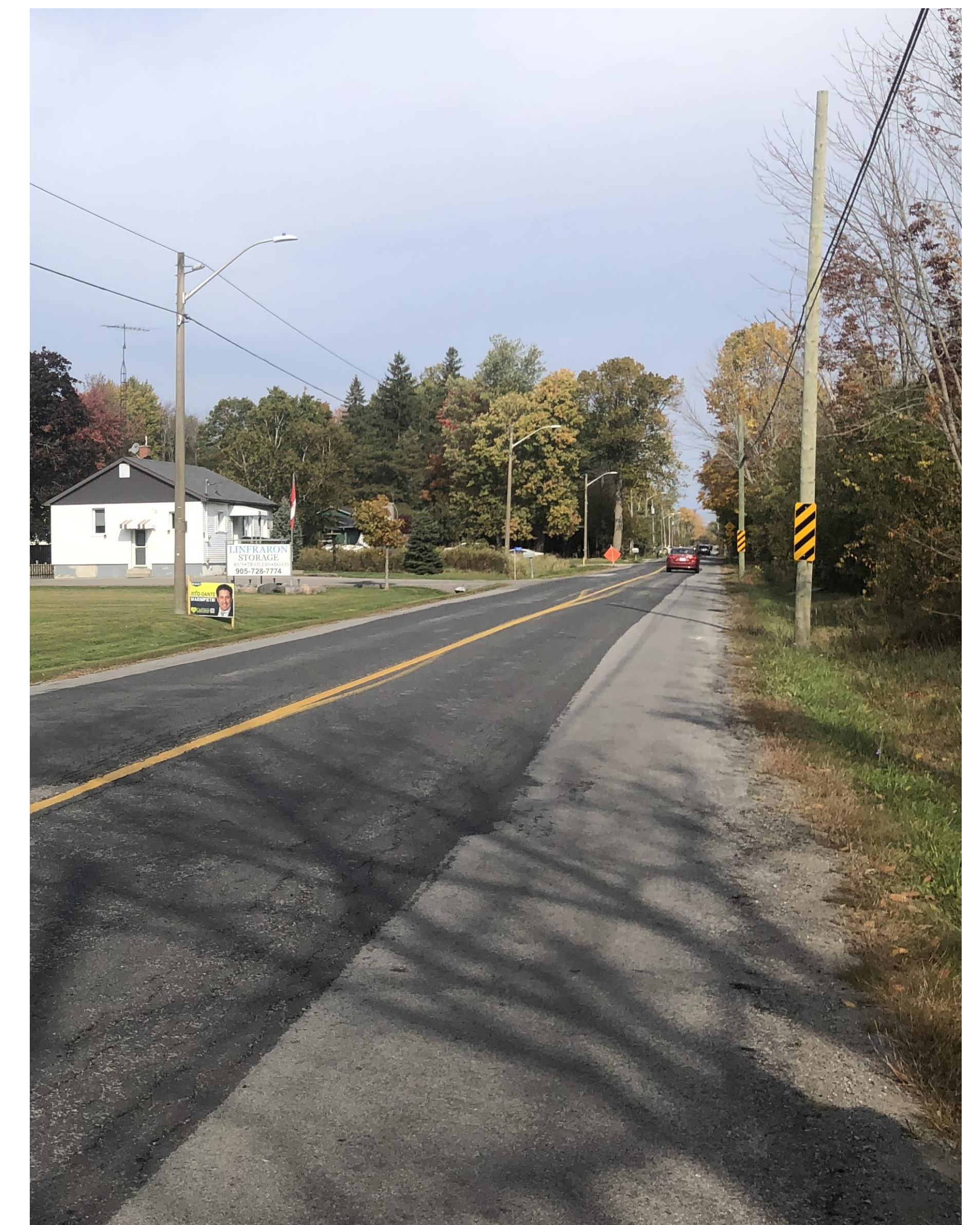
Stevenson Road North - Looking North
