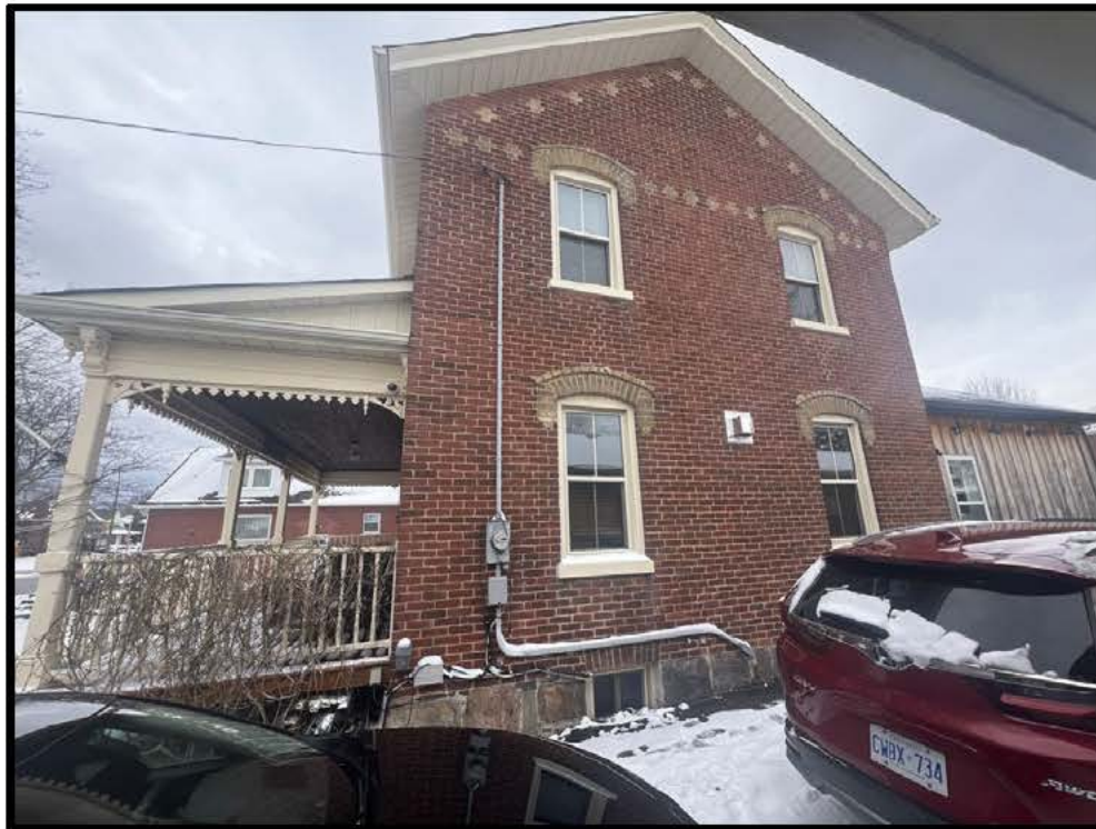
Image 8: East Elevation of 442 King Street East (Photo taken February 16, 2024; Facing West)
