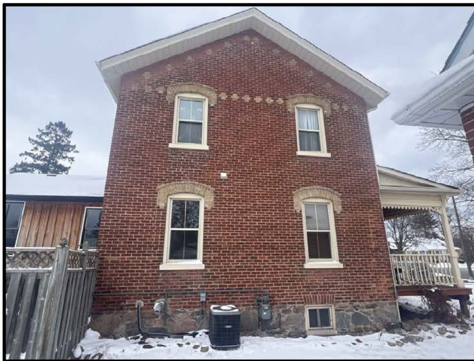
Image 3: West Elevation of 442 King Street East (Photo taken February 16, 2024; Facing East)
