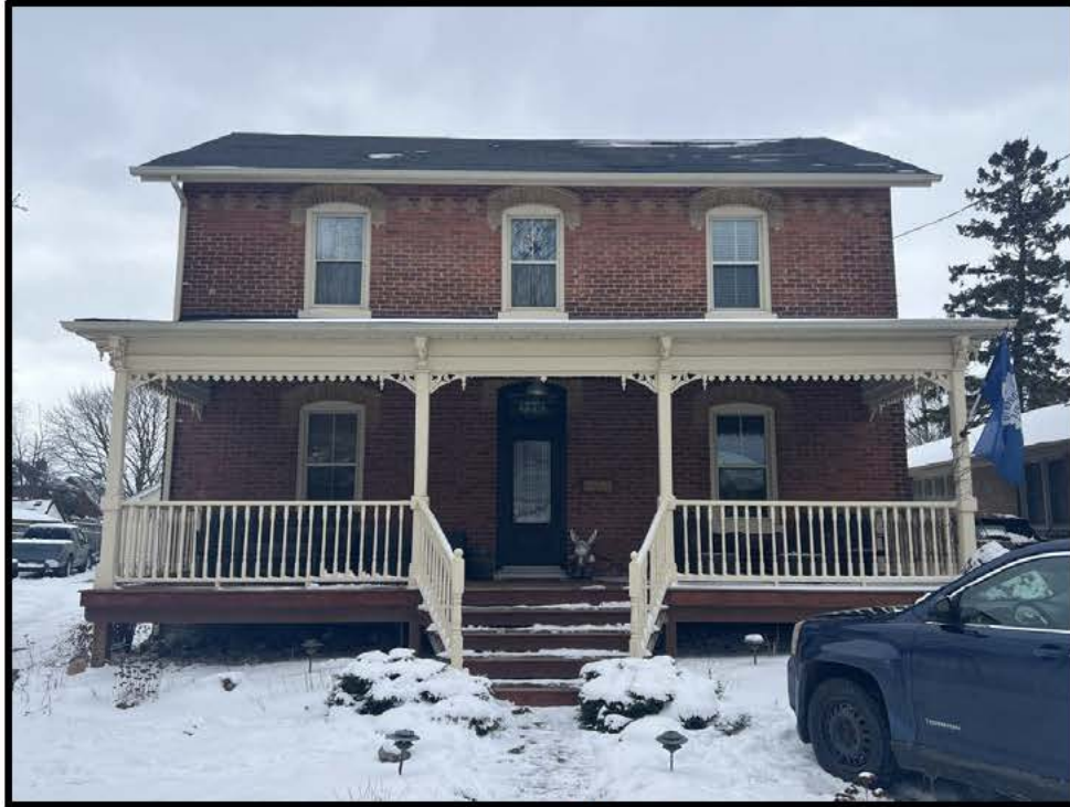
Image 1: Façade of 442 King Street East (Photo taken February 16, 2024; Facing North)
